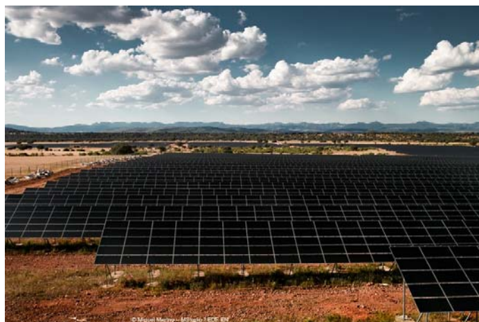
Valdecaballeros (11.4 MWp in Spain)
